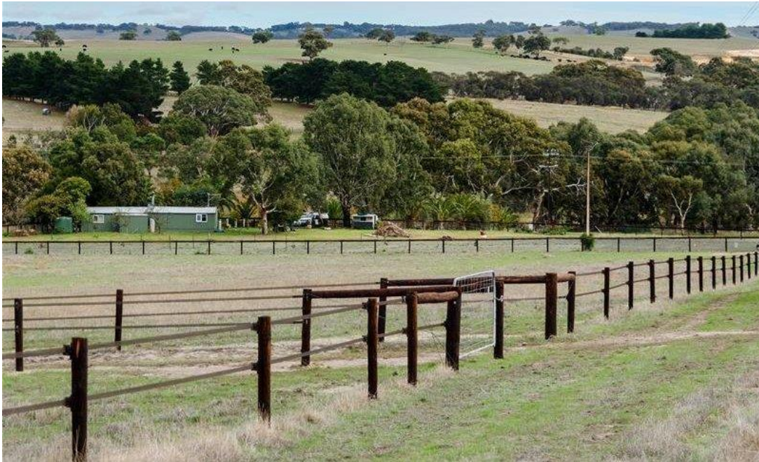
An example of two tape runs using 40mm brown electric fence tape on wooden posts set five metres apart.
